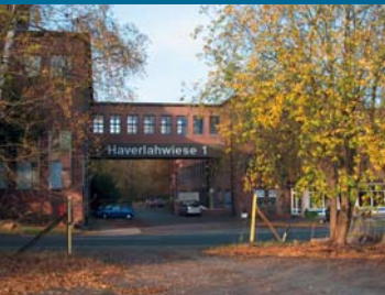
Hall for the payment of workers (“Lohnhalle”)
